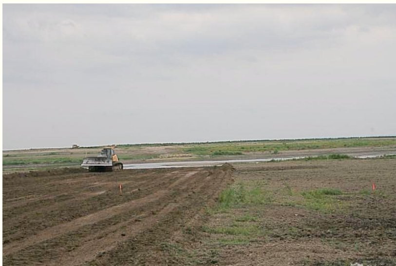
A bulldozer working in Cell 5AB
