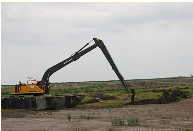
A pontoon excavator creating a tidal channel
